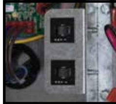
Flow center and desuperheater use breakers instead of fuses, making service and repair faster
