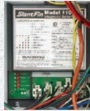
The electronic control optimizes the operation of the Victory VSPH boiler. It monitors the status of boiler components and controls the sequence of operation, indicator lights verify normal operation and provide diagnostic information.
