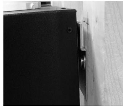
Figure 5 –Boiler Mounted to Bracket
