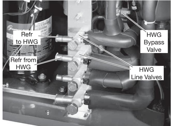
Figure 21b: Remote HWG Module
